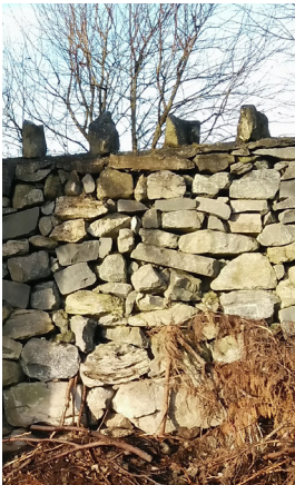
Stone boundary walls onsite
